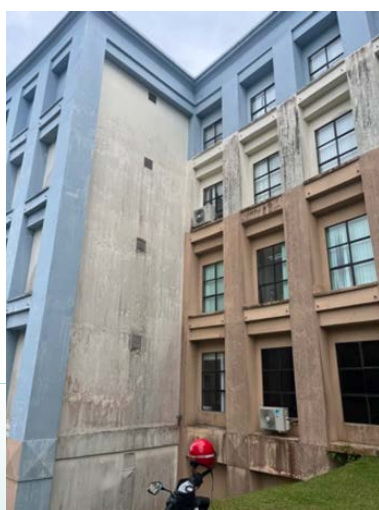
Figure 2.12: Chancellery building with natural ventilation outlets
