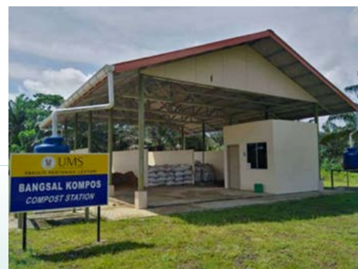
Figure 2.22: Composting station at UMS Sandakan Branch Campus
