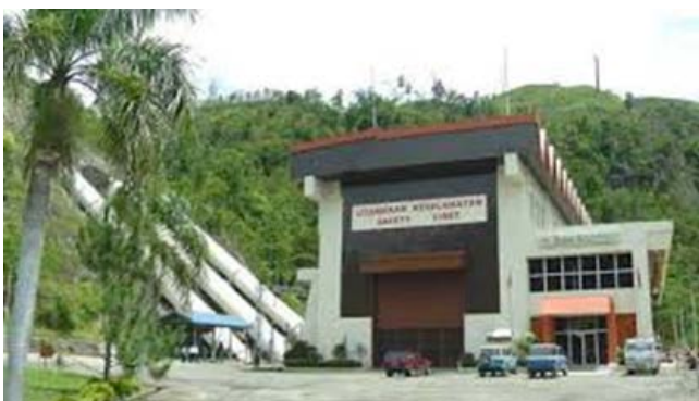
Figure 2.7: Sabah hydro power plant in the district of Tenom
