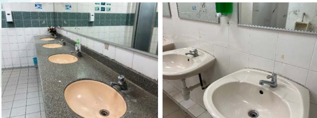
Figure 2.30: Push button type faucets and low-flow ceramic cartridge type faucets
