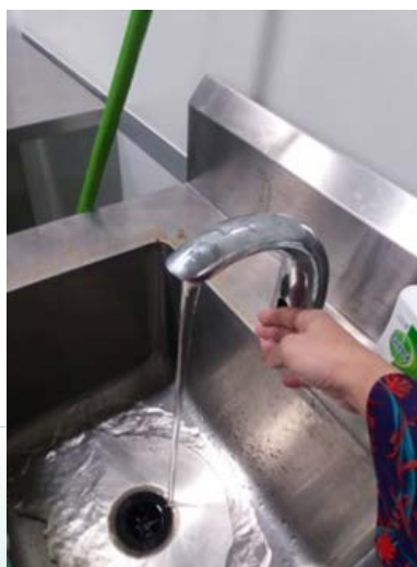
Figure 2.29: Sensor-embedded faucets
