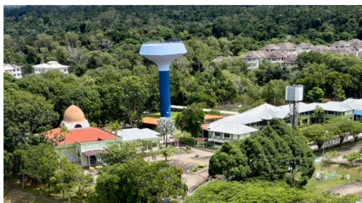
Figure 2.31: A treated water tower located on UMS Labuan Branch Campus.
