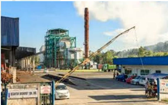
Figure 2.4: Sabah's biomass energy generation plant located in the district of Sandakan
