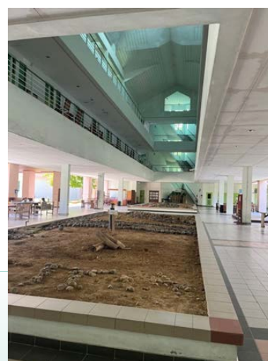
Figure 2.13: Faculty of Tropical Forestry main building with large indoor atrium
