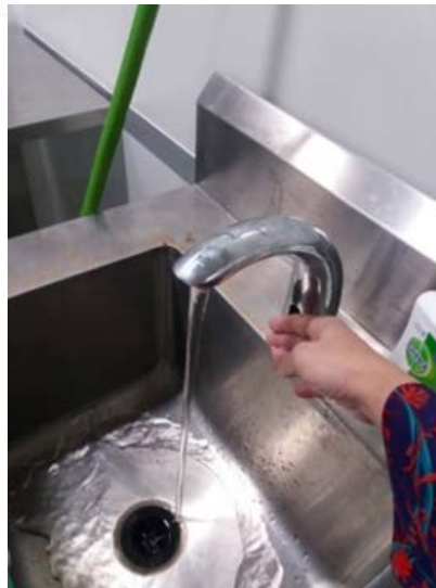
Figure 2.29: Sensor-embedded faucets
