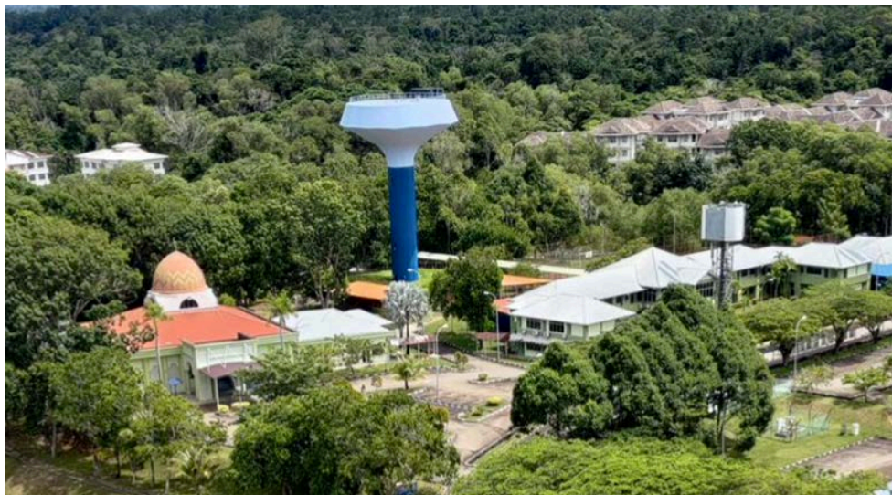
Figure 2.33: A treated water tower located on UMS Labuan Branch Campus.
