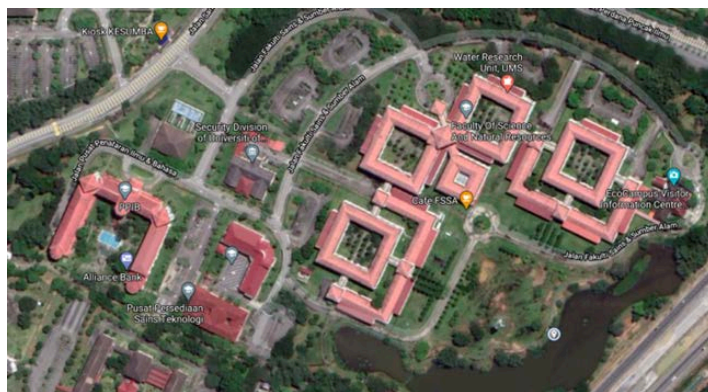
Figure 2.11: Faculty of Science and Natural Resources building complex with large central atriums
