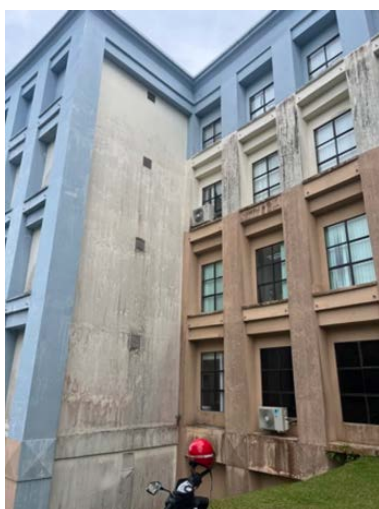
Figure 2.12: Chancellery building with natural ventilation outlets
