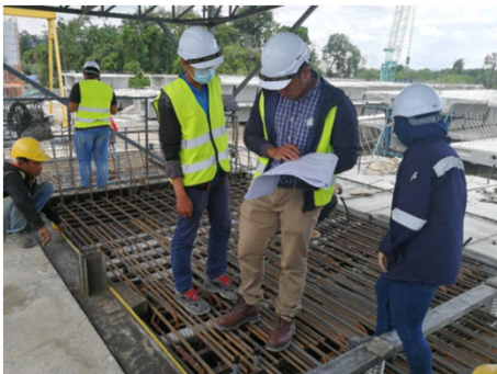
Student checking actual measurement against drawing during pre-concreting of segmental box girder (Picture Courtesy of Dayang Nur Hidayati, HK01)
